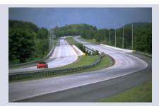
With life cycles of over 40 years, concrete roads offer benefits such as less maintenance and lower rolling resistance (less fuel consumption) when compared to asphalt roads.
