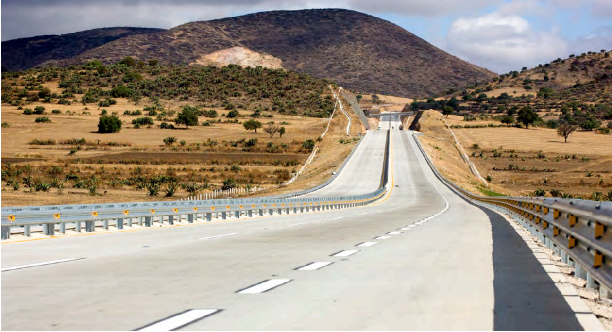
Arco Norte Highway, Mexico
