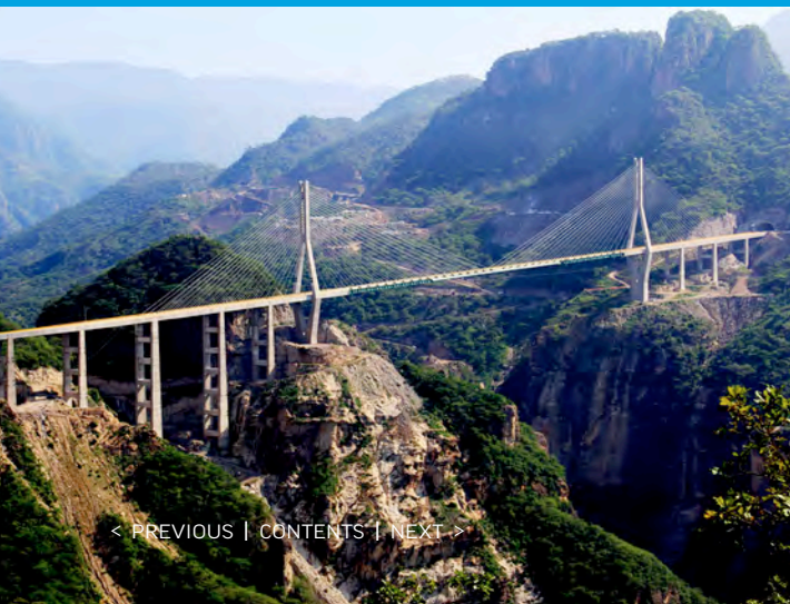
Baluarte Bridge, Mexico
